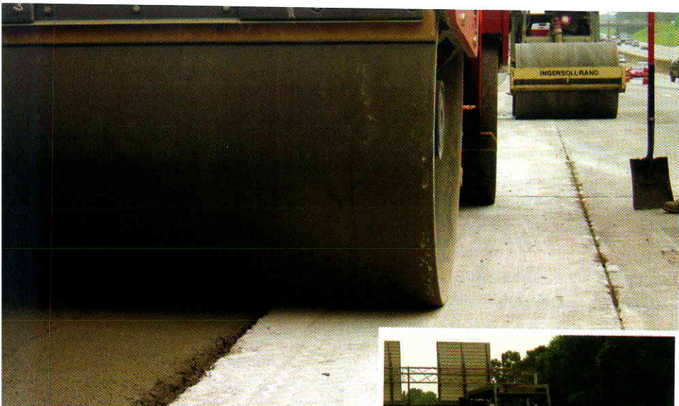
Above & Right: After placement, the RCC was immediately rolled to 98-percent density. Here, a Hamm roller – one of two rollers used on the project – compacts the RCC.
